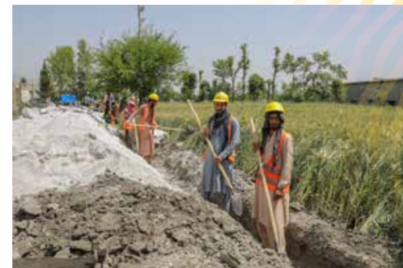
Canal rehabilitation in Nangarhar province, Eastern region
