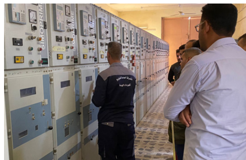
O&M CDAs delivered onsite training to the Diyala Electricity Department.
