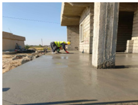
Civil work in progress- casting concrete for Floor
