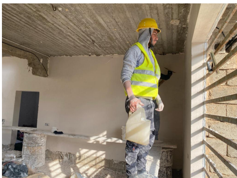
Civil work in progress- plastering
