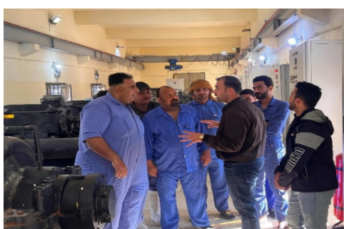
O&M CDAs visited Big Ramadi Water Project in Anbar governorate to discuss operational challenges. Operators identified maintenance issues like chlorination devices, horizontal pumps, air-conditioning split units, and RO filters. UNDP Engineers and O&M provided expert guidance, equipping operators with the necessary skills for periodic maintenance and project reliability.
