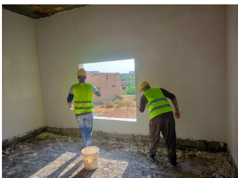
Civil work in progress- painting.
