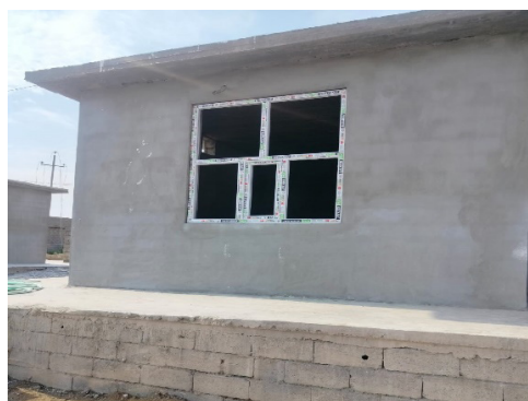
Civil work in progress- cement plastering.
