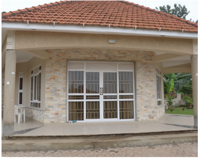
House finished with stone wall tiles by Kyogo Mazinga Company, Uganda
