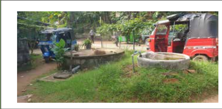
Biogas Unit in Karapitiya Hospital
