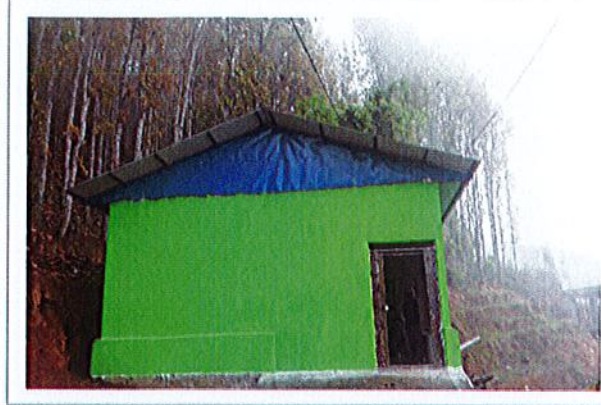
Women Cooperative Building -Dhading
