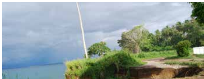
The coastal road to Pokili WMA has been eroded and the coastline has retreated many metres, threatening houses and infrastructure © Ann Peterson/Protected Area Solutions
