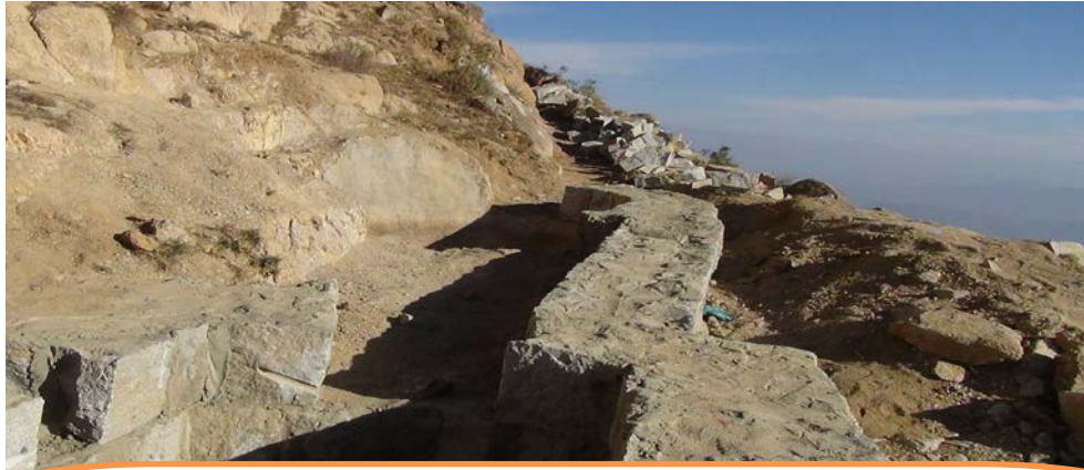
Closed rocky tank Channels After the intervention of the project Jabal Al-U'lia
