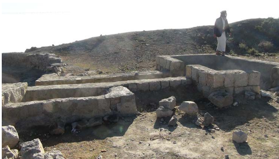
open rocky tank Channels(filter holes) After the intervention of the project Jabal Al-U'lia Manakha
