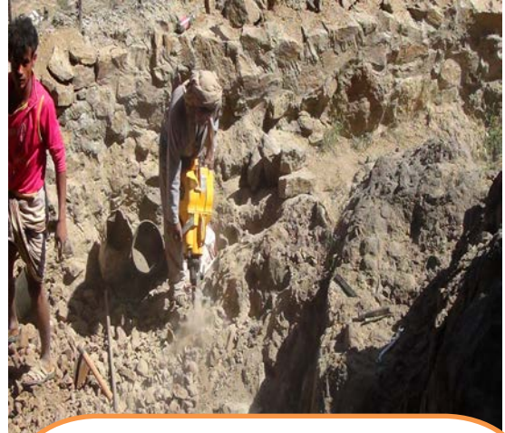
Drink water- Rocky tank before project intervention – Al-saawd Mankha
