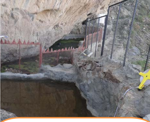
Drink water- Rocky tank after project intervention – Al-saawd Mankha
